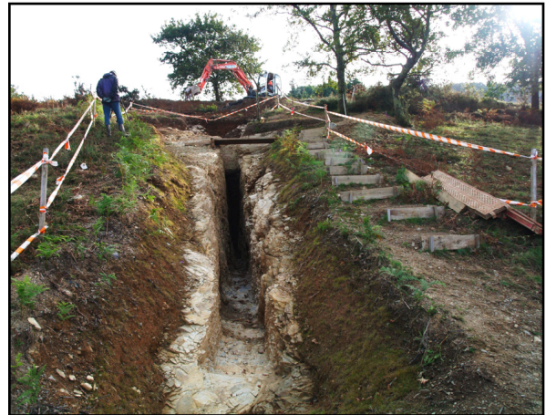
FIGURE 1. Arditurri 3, entrance of the tilted gallery.
