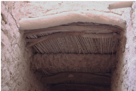
Figure 4. Covering system made of half date palm trunk, tamarix beams and date palm midribs (Al-'Ula, Saudi Arabia, © C. Bouchaud).
